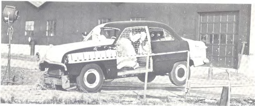
Early crash simulation device at CAL showed action of articulated dummies
